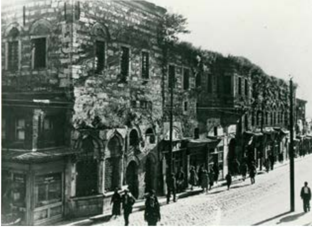
Figure 5. Istanbul. Simkeşhane, 20 th century. Ataturk Library, Husrev Tayla Archive, Accession N. FOTO_019084. The fountain can be seen on the corner of the building facing the street on the far left. The types of shops on the ground floor, the poor condition of the units on the first floor and the heavy vegetation on the roof suggest that the building was already in a poor condition in this period and the simkeş craftsmanship had already waned. The shop on the bottom left of the photograph reads “ manav ”, which means greengrocer. The clothes of pedestrians (men in suits with hats, women without headscarves and with skirts) and the use of Latin script for “ manav ” indicate the photo was taken after 1928. A tram line is also visible on the street. This was constructed in 1914 in the second constitutional era of the Ottoman Empire (1914-1918).
