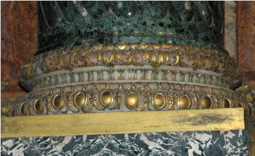
Figure 6. Santa Teresa Chapel, detail of column bases (photo by D.R. Marshall, 2004).
