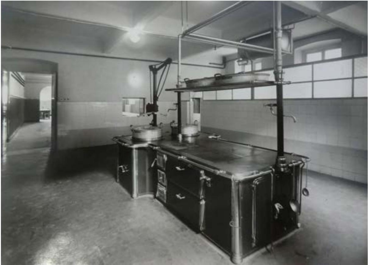
Figure 23. Montelucio di Roio (AQ), Colony IX Maggio. The electric stove for large communities, sponsored by the Unione Esercizi Elettrici on the pattern of the one already in use in Ancona's Psychiatric Hospital after the 1930 earthquake (Rome, AIGMF, ENAGM, *Colonia Montana di Rojo*, 1937-1961).
