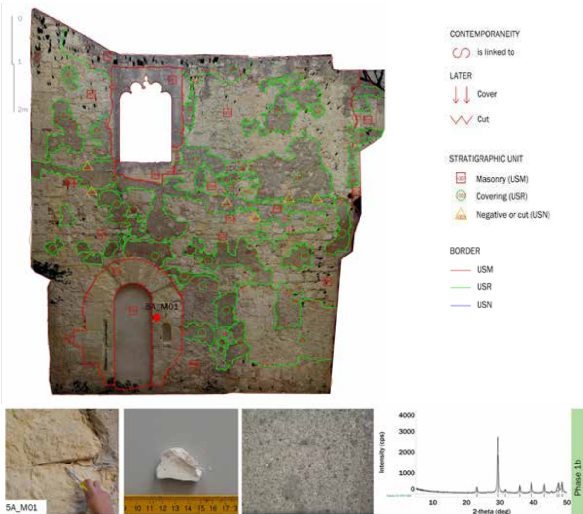
Figure 27. Example of stratigraphic analysis of a masonry of the convent and the mineral-petrographic analysis of one of the twenty sample of mortar (5A_M01). From the left: sampling localisation, macroscopic and microscopic view (2.5x), and diffractometry (elaboration by E. Pilia).
