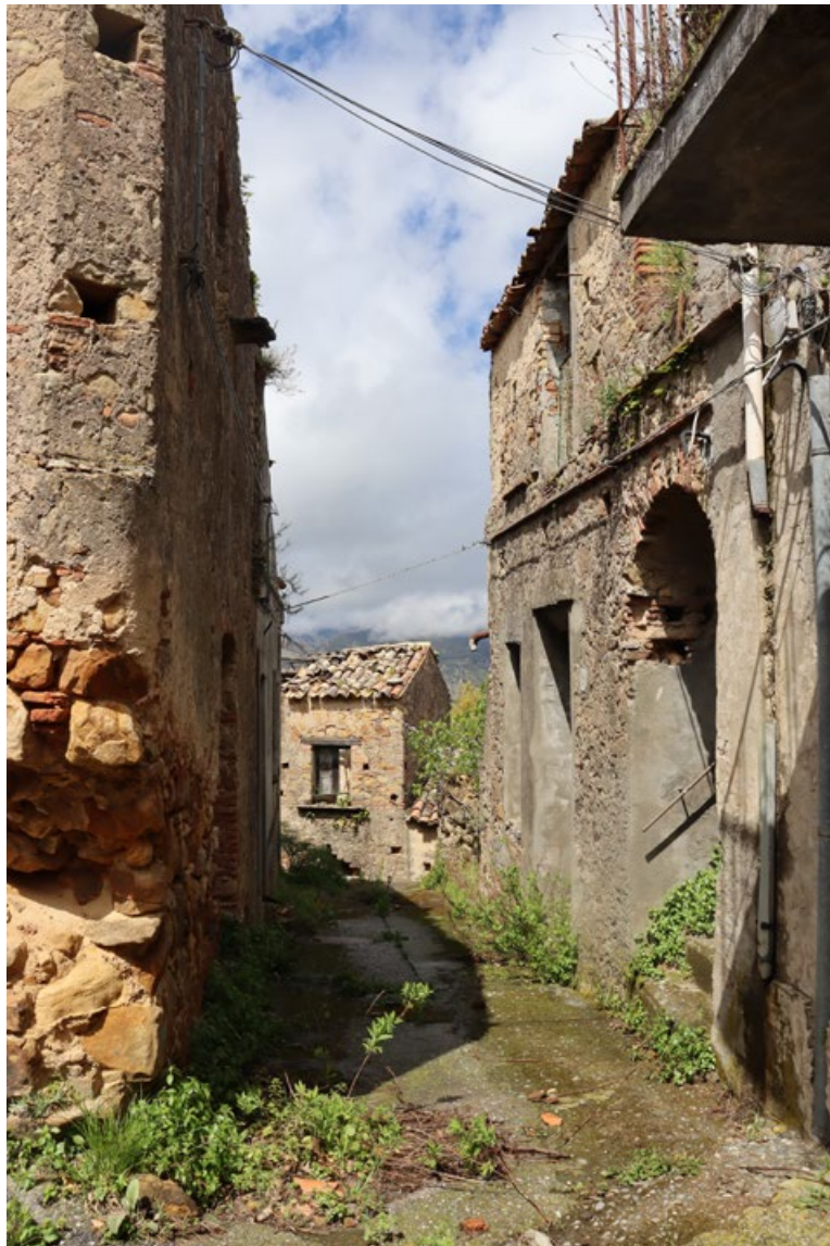
Figure 9. Ferruzzano Superiore, buildings in vico Cavour (photo C. Valiante, 2023).
