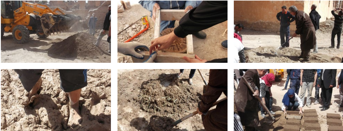
Figures 3a-f. The stages of adobe production during the restoration of the ksar of Lichana in 2015 (photos S. Zerari, V. Pace, L. Sriti, 2015).
