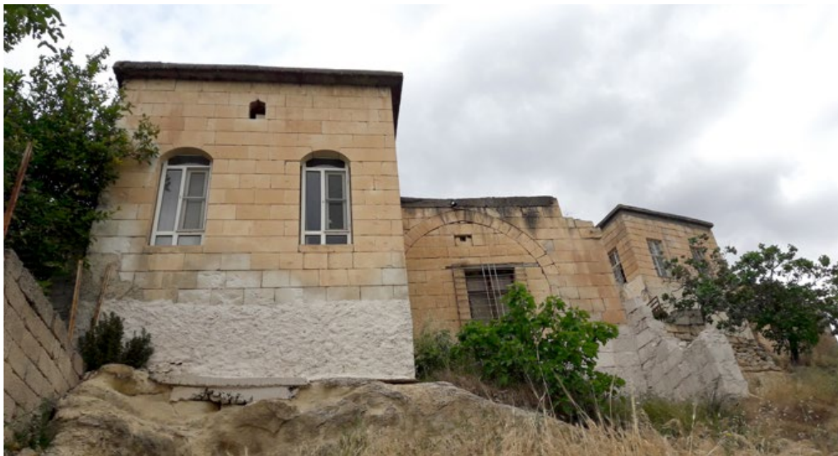
Figure 5. Examples from vernacular architecture in Old Halfeti (photo A. Özmen, 2018).
