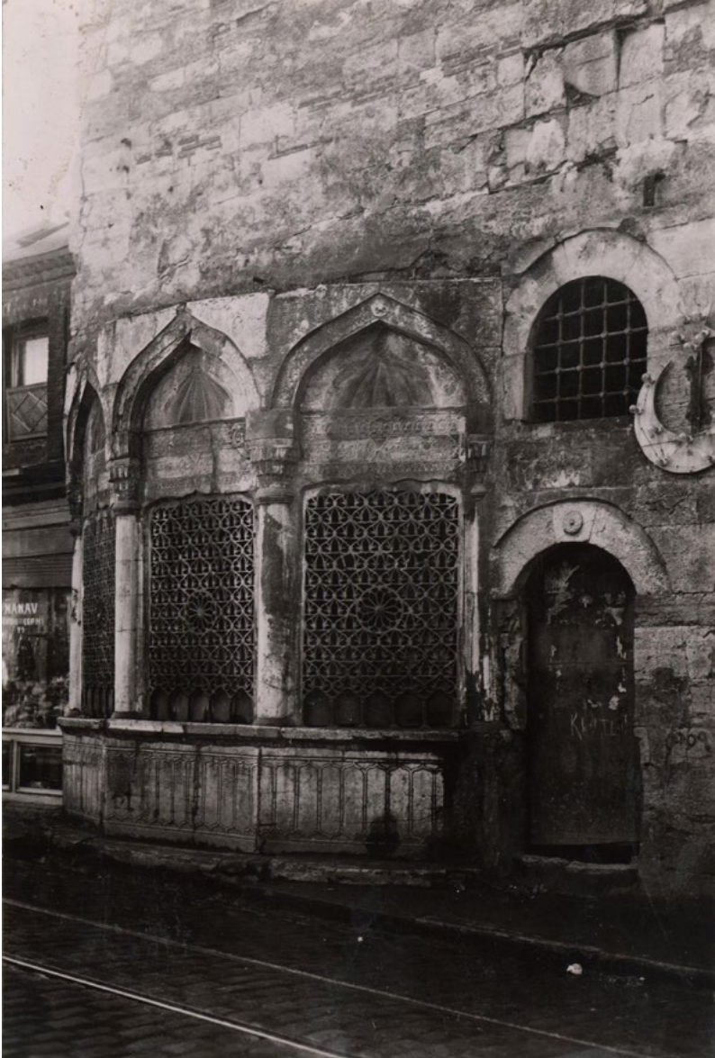
Figure 6. Istanbul. The fountain of Simkeşhane in the 40s of the 19th century, Salt Research Archive, Archive No. TASUH0909 ( https://archives.saltresearch.org/handle/123456789/74329 , access June 15 th 2019). Construction of water elements (i.e. fountains) with ornamented surfaces by Ottoman women patrons in the 17 th century is a common feature of the Tulip period, which marks the beginning of European influence in the Ottoman urban texture. Moreover, it is noteworthy that also in the Forum Tauri there a nymphaeum.
