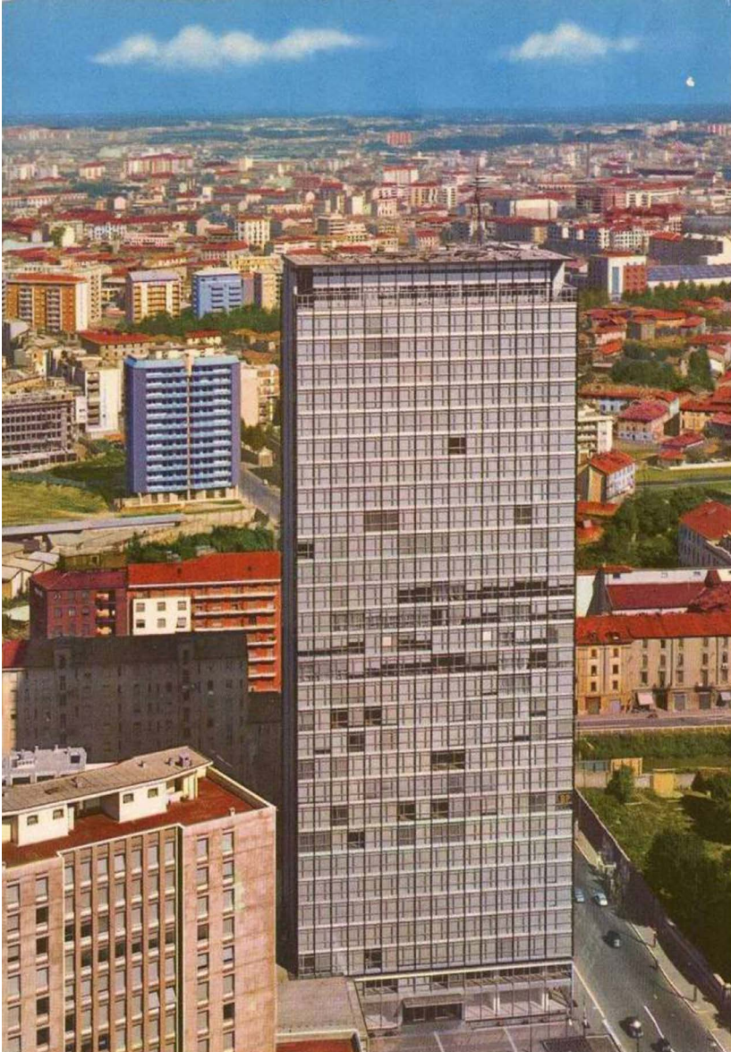
Figure 2. Milan, Galfa Tower façade with curtains, view from Pirelli Tower rooftop (1960s-postcard, collection of the authors).
