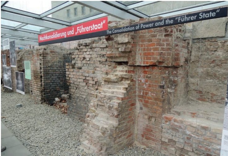
From top, figures 20-21. Berlin. Views of Topography of Terror (photo by F. Murè).
