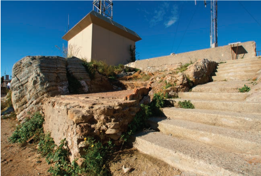
On the left and on the next page, figures 22-23. Turó de la Rovira - Barcelona. Views of Els Canons area after the restoration in 2011 (photo by F. Aiello - www.francescoaiellophotographer.com ).
