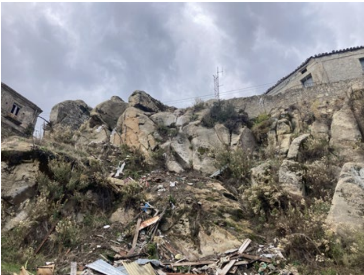
On the previous and on this page, figures 13-16. Ferruzzano, Reggio Calabria. The rocky outcrop where Ferruzzano is located shows a prevalent division according to vertical planes and prisms (photos N. Sulfaro, 2023).
