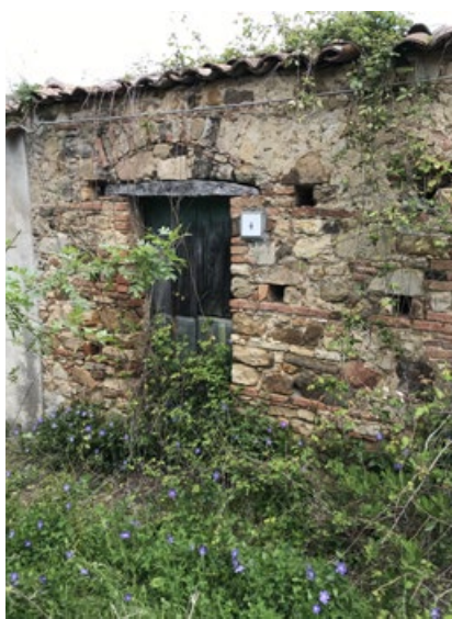
Figures 24-29. Ferruzzano, Reggio Calabria (photos N. Sulfaro, 2023).
